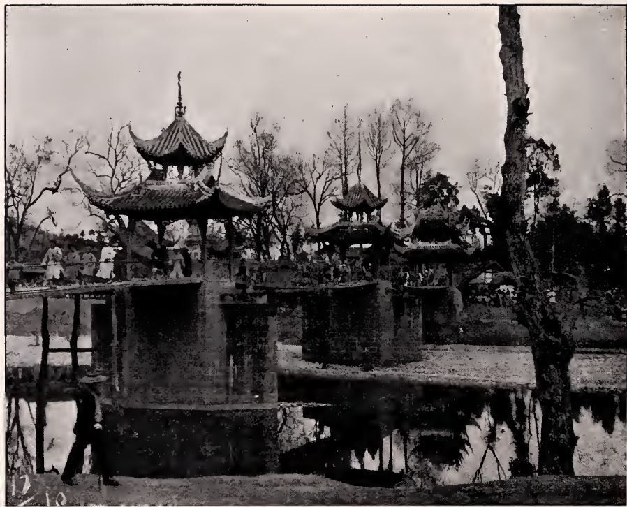
Bridge on the Chengtu-Tibetan Road, crossing irrigation channel— partly natural, partly artificial.
